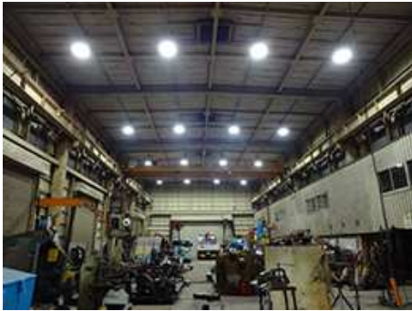
Kikuchi Industry (After Construction)
